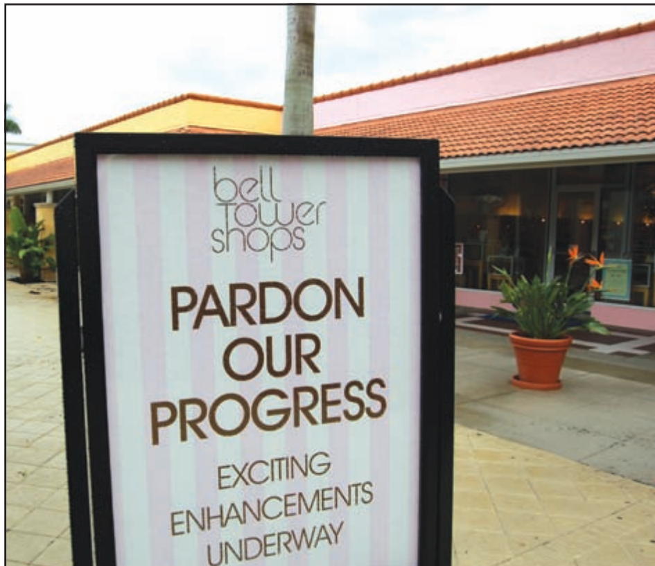
The first phase of the renovation project at the Bell Tower Shops is under way and will cost about $2 million.
