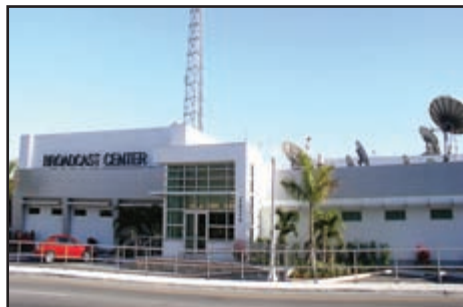
The Fort Myers Broadcasting building
