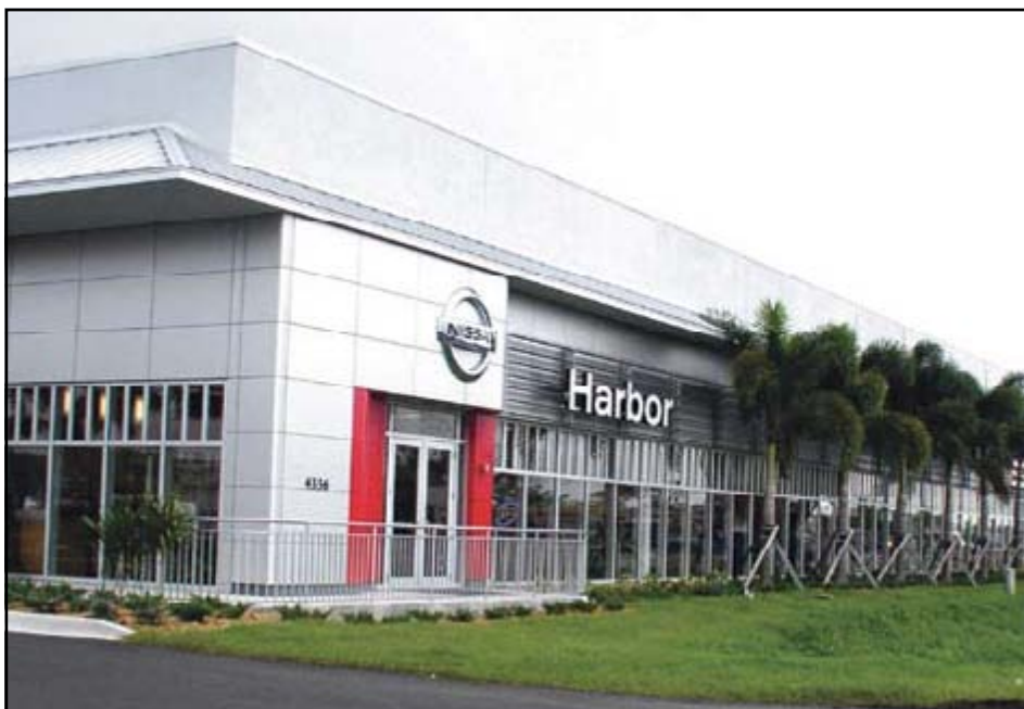
Owen-Ames-Kimball Company recently completed construction of the new Harbor Nissan in Port Charlotte.
