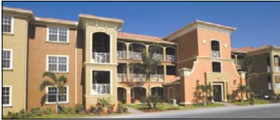
PHOTO COURTESY ENGLE HOMES
